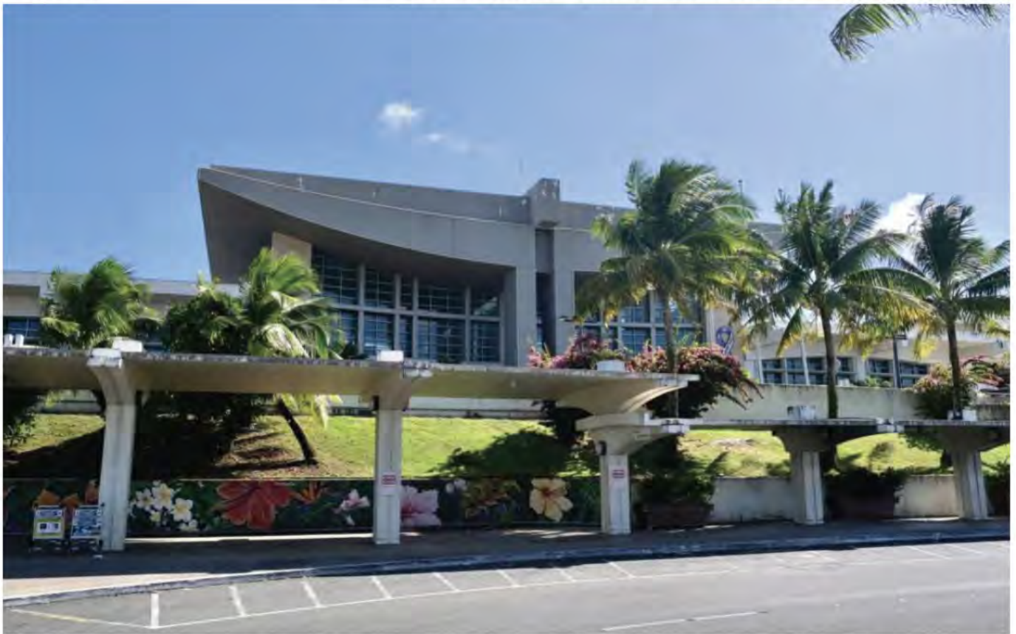
GIAA: The Antonio B. Won Pat International Airport in Tamuning is shown on Thursday, Jan. 16, 2025. Frank San Nicolas/The Guam Daily Post
