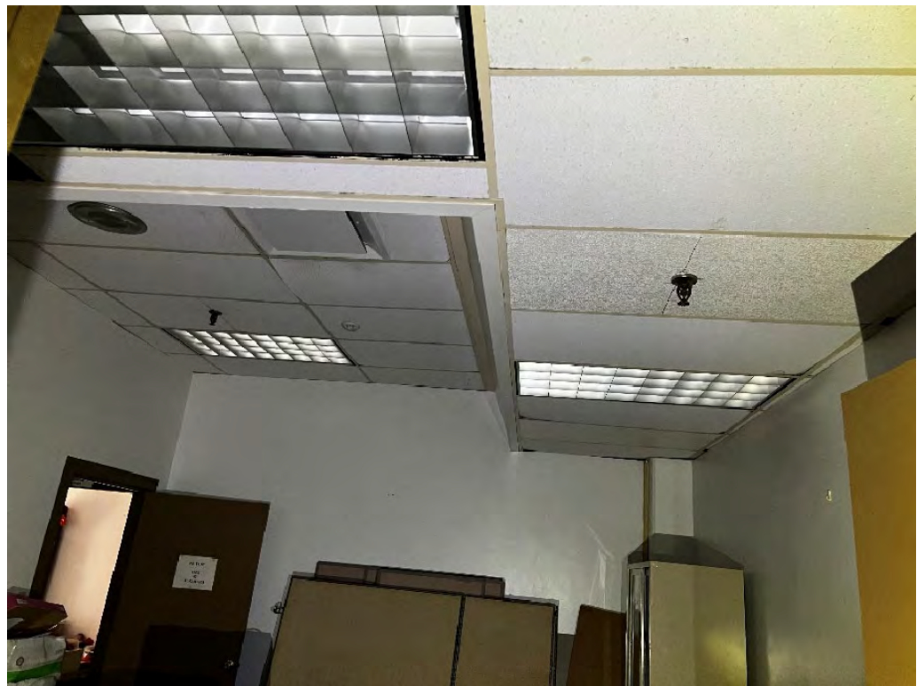
PHOTO #9 – EXISTING LIGHT FIXTURES
