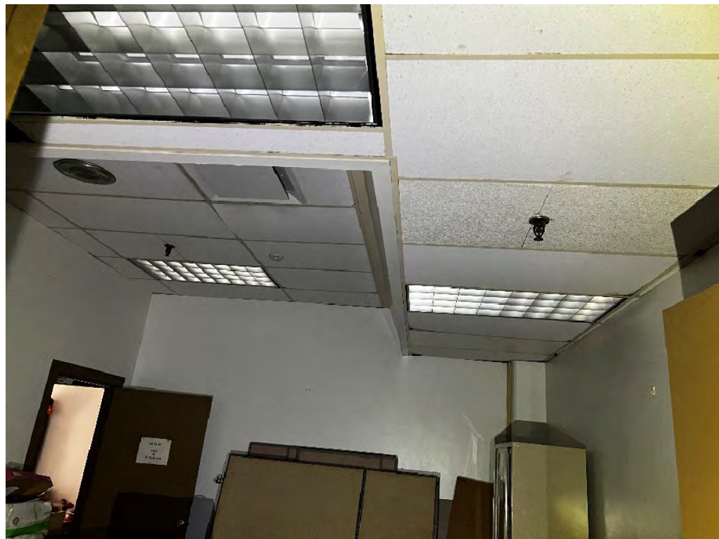
PHOTO #9 – EXISTING LIGHT FIXTURES
